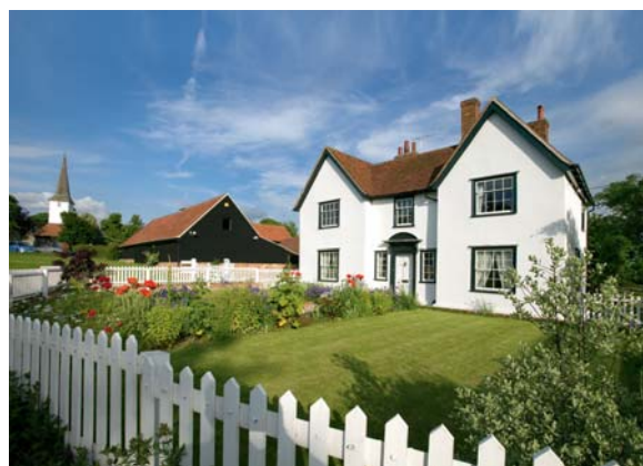
Bellmans Farm - after renovation
