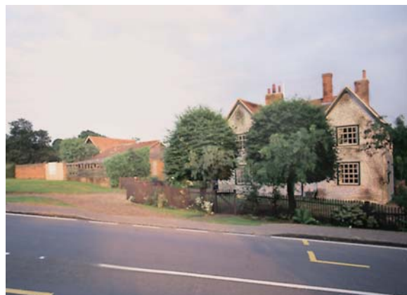
Bellmans Farm - before renovation
