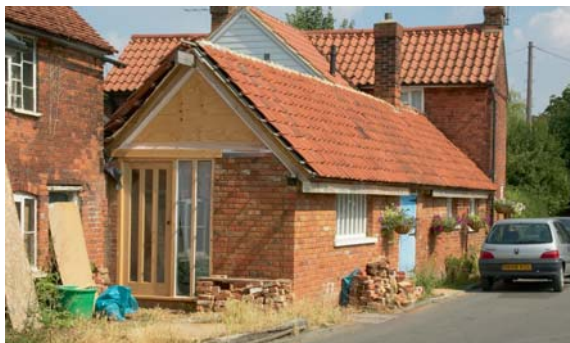
Restoration in progress
