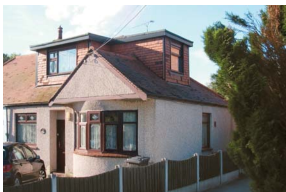
Poor example of additional dormers
